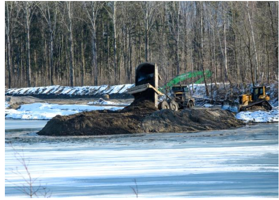
Figure 19: A long reach excavator used for shaping the shallows at Ausee (left). Dumping into Ausee was a challenge for the construction companies owing to difficult weather and soil conditions (right, photos: Ragger/REVITAL).
