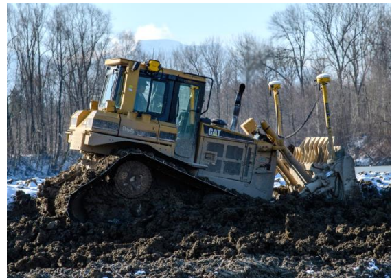
Figure 18: Sand and gravel removed from floodplain lowering areas and transported to Ausee using dump trucks (left), GPS-equipped bulldozers at work at Ausee (right, photos: Ragger/REVITAL).
