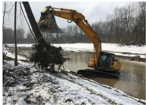
Figure 20: Large oxbow lake created in extant gravel at Reitbach (floodplain lowering area 4 - VA4, left, photo: Ragger/REVITAL), placement of rootstocks to structure the Reitbach (right, photo: Zauner/ezb)
