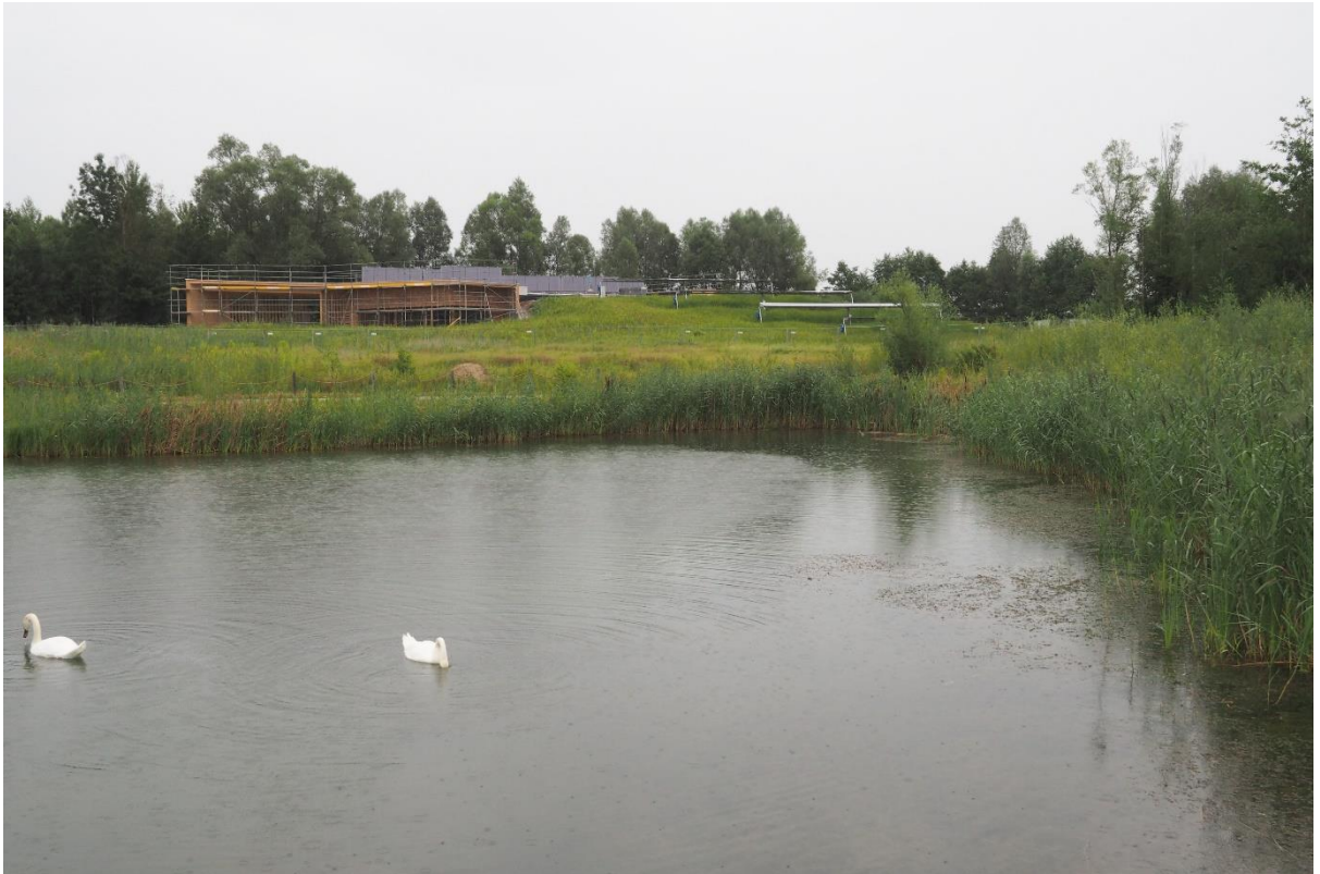
Figure 8: The new riparian forest workshop “Auenwerkstatt” in the Weitwörther Au under construction (Photo: Riehl)
