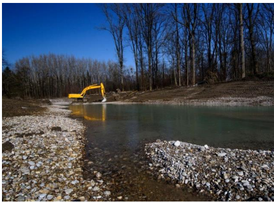
Figure 20: Large oxbow lake created in extant gravel at Reitbach (floodplain lowering area 4 - VA4, left, photo: Ragger/REVITAL), placement of rootstocks to structure the Reitbach (right, photo: Zauner/ezb)
