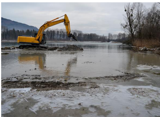
Figure 21: Remaining works at Ausee began on 17/12/2018. These are small-scale modifications, primarily to create shallows. (Photos: Zauner/ezb)
