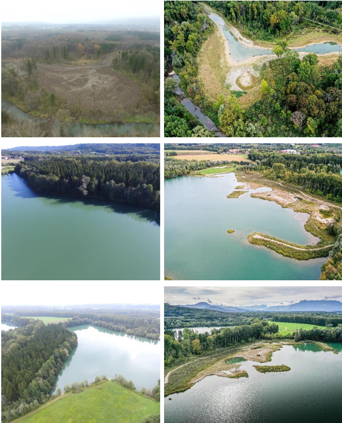
Figure 23: Before (2017) - after (2019) of the Reitbach action areas (left to right), showing floodplain lowering area VA4 (top) and the Ausee (middle and bottom, photos: REVITAL)
