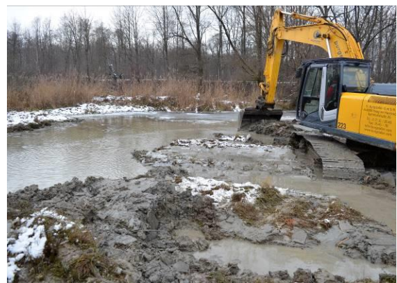
Figure 21: Remaining works at Ausee began on 17/12/2018. These are small-scale modifications, primarily to create shallows. (Photos: Zauner/ezb)
