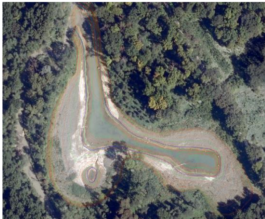
Figure 13: Planned elevation profile (coloured lines) and actually implemented measures match perfectly. (Ortho-photo: Province of Salzburg)
