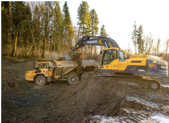
Figure 18: Sand and gravel removed from floodplain lowering areas and transported to Ausee using dump trucks (left), GPS-equipped bulldozers at work at Ausee (right, photos: Ragger/REVITAL).
