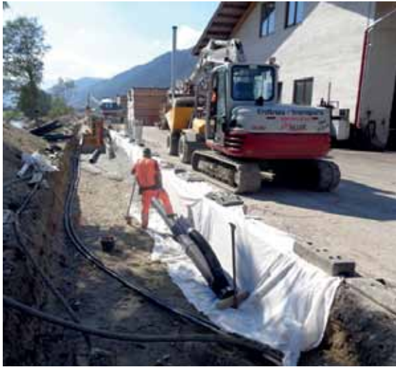
HWS-Mauer in Bau ....
